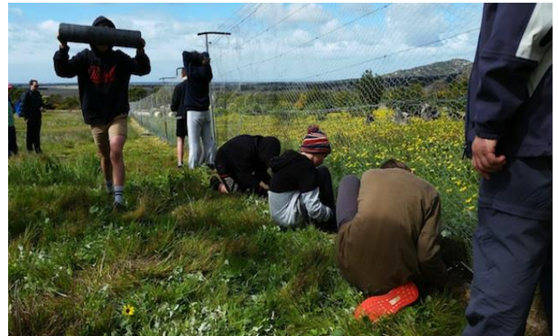
Installing rabbit proof fence
